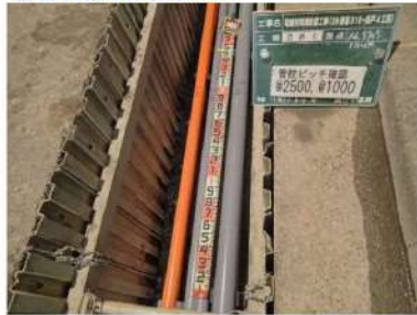
⑪管台設置間隔2.5m
